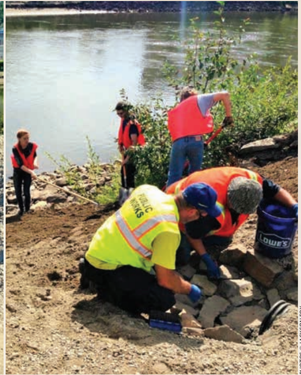
With the concrete chute removed, volunteers worked diligently to rehabilitate the river bank with topsoil, grass seed and live willows.
