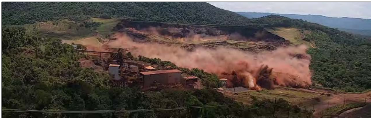
Figure 4. Tailings dam failure at Brumadinho, Brazil, 18 seconds after the initiation of the failure
