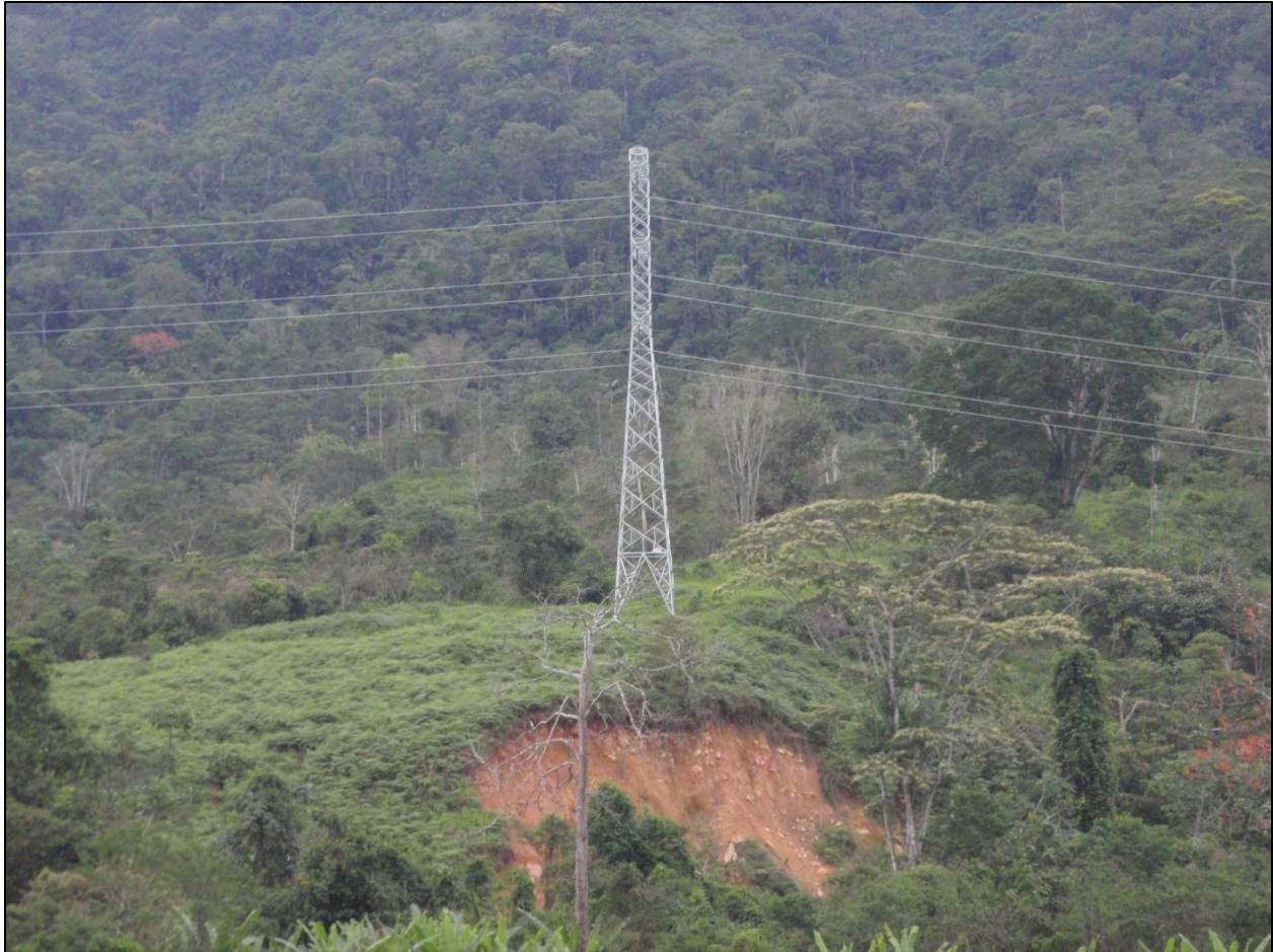
Figure 15. The high erosion rate in the project area is indicated by the landslide scar below a transmission tower on the north bank of the Rio Quimi (see Fig. 11), opposite the Quimi tailings dam. Photo taken by the author on November 6, 2018.
