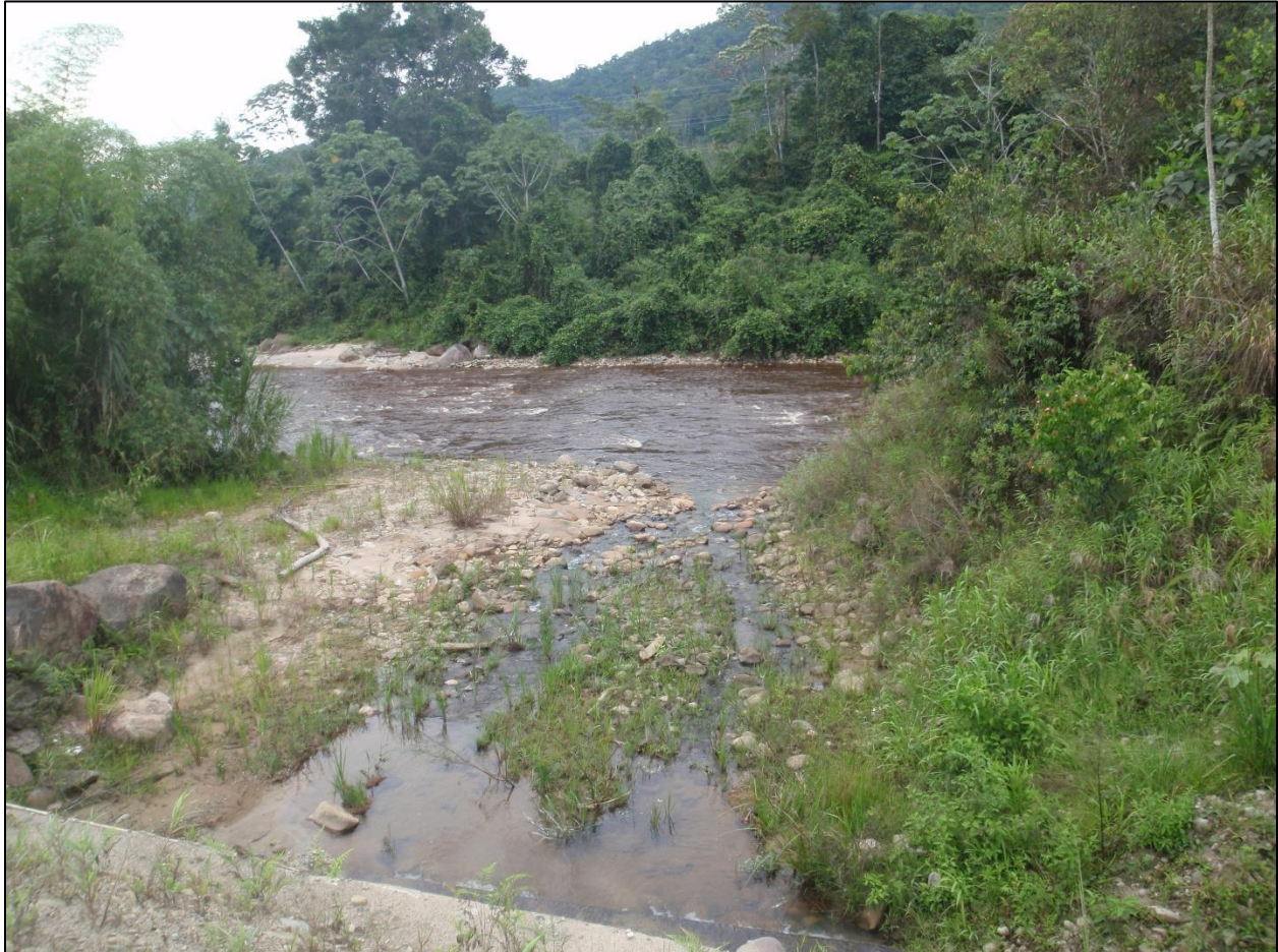
Figure 19b. The pipe from the sedimentation ponds discharges directly into the Rio Quimi. Photo taken by the author on November 6, 2018.
