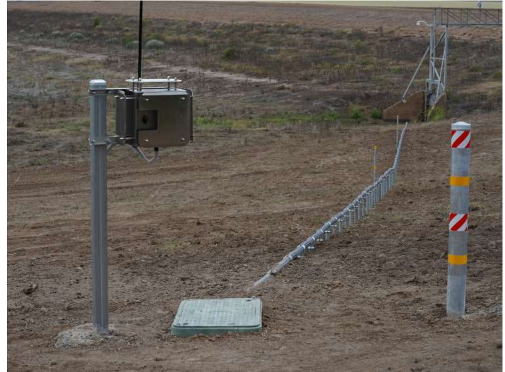
Image: of installed submersible embankment.
