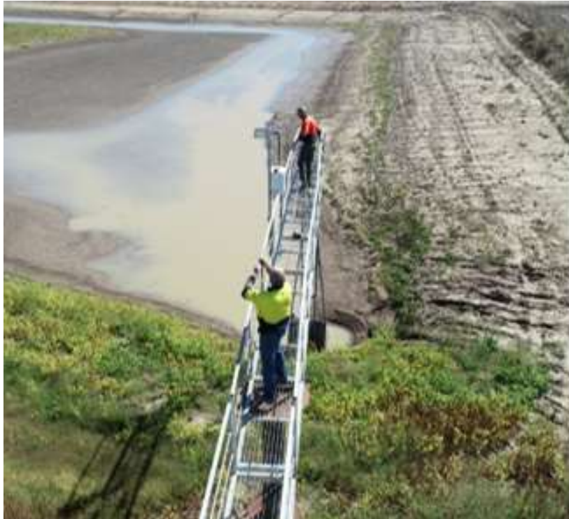
Image: Installation of submersible (elevated platform) meter.
