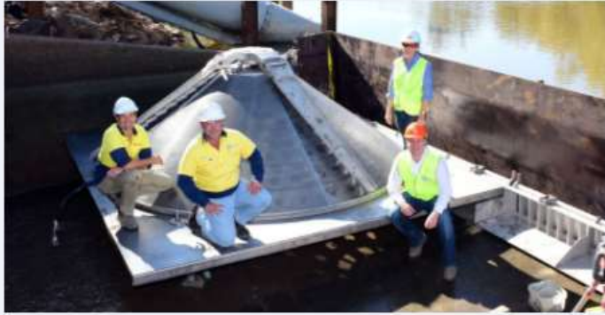
Trangie-Nevertire Irrigation Scheme
