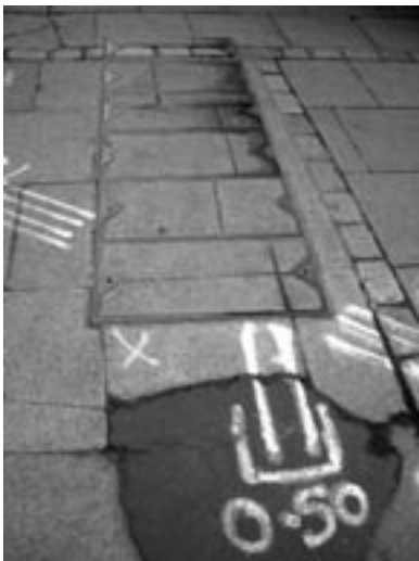
Figure 59: Revealing hidden infrastructure Survey lines showing the multiple networks beneath pavements, Leith Walk, Edinburgh
