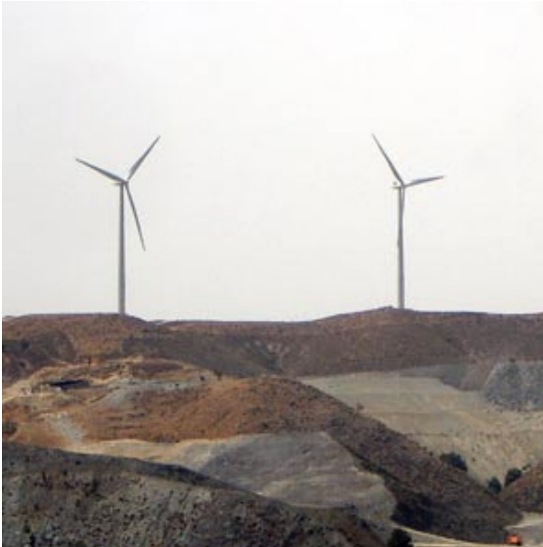
Figure 44: Windfarm. Granada, Spain
