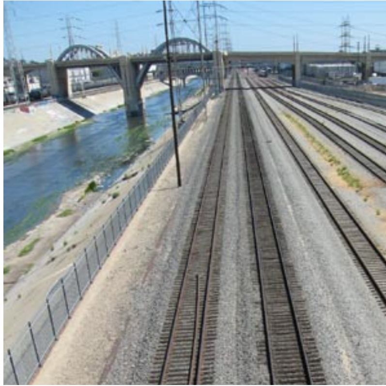
Figure 40: LA River, Bridge and Tracks
