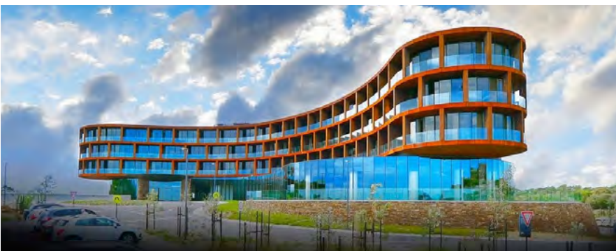
RACV Cape Schank Resort - A Kane project
