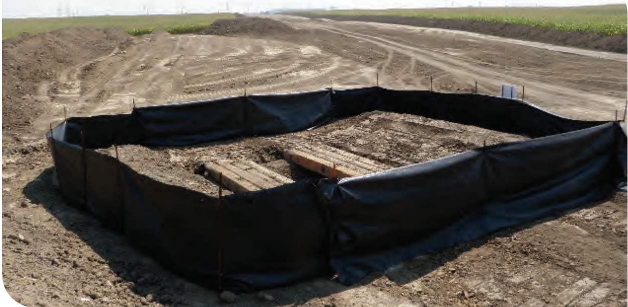
Cleaning station at construction site.
