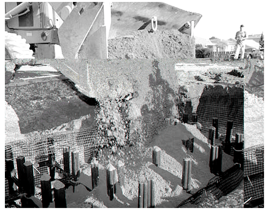
Figure 5 Installing absorbent soil in cells
