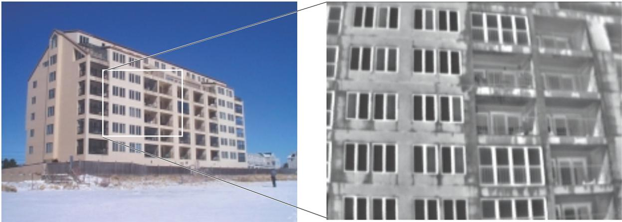
**Figure 10.** Rainwater entering through cracks in EIFS can lead to mold growth. IR images show moisture accumulation here.
