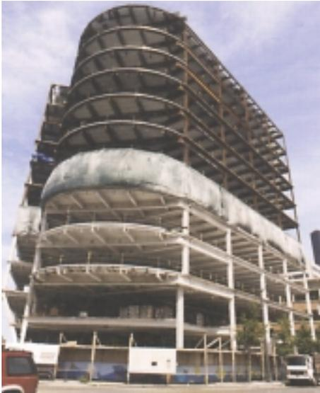
**Figure 5. In high-rise construction, water from upper stories can wet lower finished floors.**
