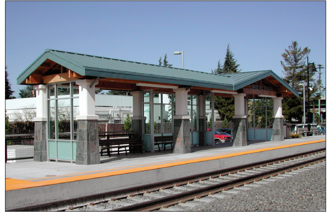
▲ Figure 3: A rail station can function with just a platform, ticket kiosk, and surface parking lot. However, a well-planned rail station can become a valuable community asset.
