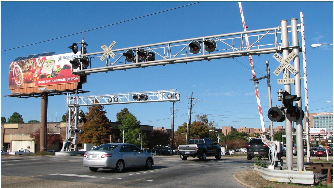
▲ Figure 7: Gates and flashing lights will be installed at all public grade crossings on the corridor.
