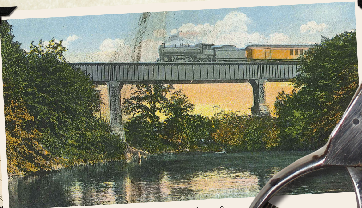
High Bridge - Train over Quinebaug River, Putnam, Conn.
