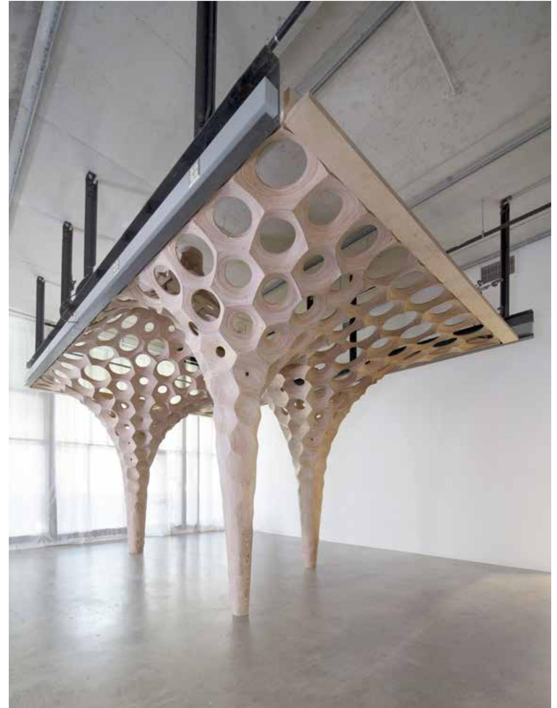
La Voûte de LeFevre is a mashup of ancient stereotomic vault construction with contemporary computation and advanced fabrication. The vault is a compression-only structure calculated through a custom simulation program to
