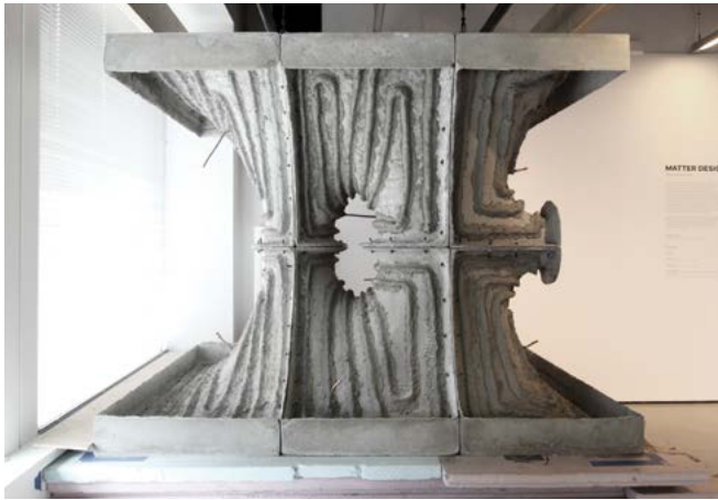
7 View of the shell back side before cladding (Clifford, 2015, © Matter Design).
