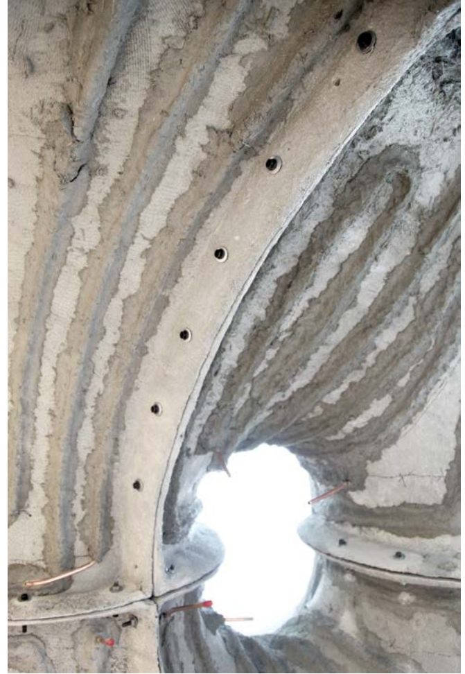
8 Detail of the assembly flanges (Clifford, 2015, © Matter Design).
