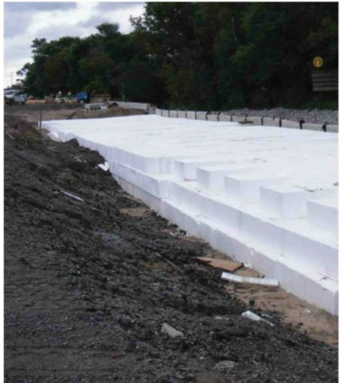
Geofoam weighs only about 1 to 3 pounds per cubic foot and is easy to place by hand.
