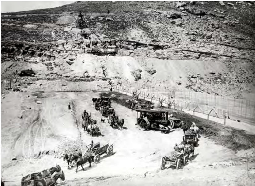
Federally funded project, Strawberry Reservoir
