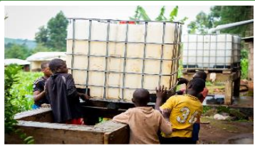
Rainwater Harvesting System Installation
