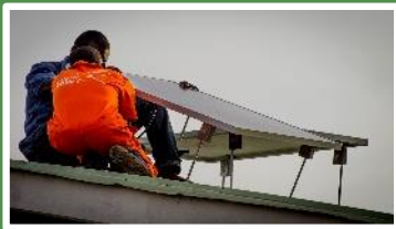
Solar Panel Installation
