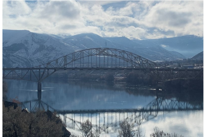
Figure 2-14: George Sellar (SR285) Bridge
