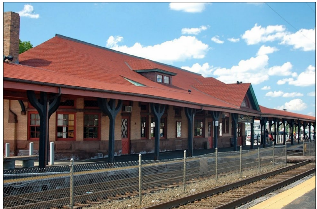
Beverly Depot is one of many stations on the line without high-level platforms, despite its substantial ridership.
