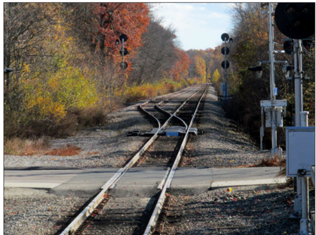
While the full lines don't require double-tracking to achieve high performance, building additional tracks in a few specific locations is key in allowing trains to pass each other.
