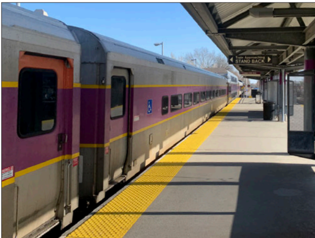
High-level platforms allow passengers to easily step off the train without climbing stairs. These are needed at the stations along the Hyannis extension.
