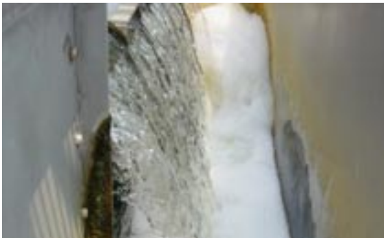
Tertiary treated water overflow at municipal WWTP.
