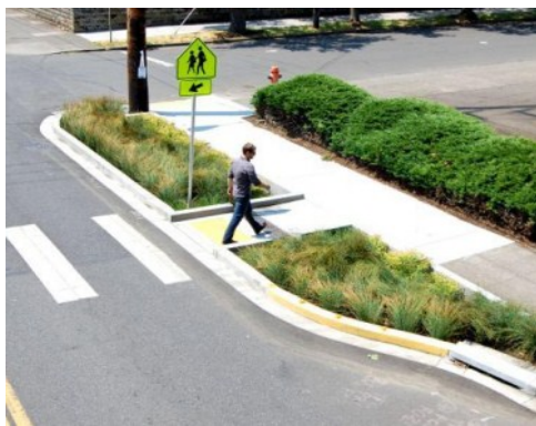
Accessible pedestrian ramps can also be integrated into the design. Source: Dave Elkin/City of Portland
