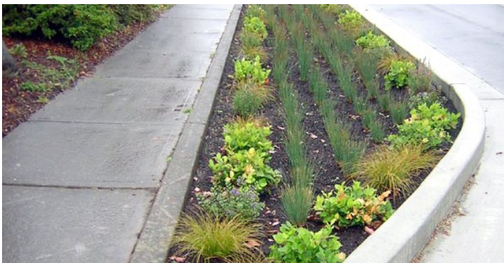
Existing curb retained while installing a bioretention along a neighborhood collector street. Source: Kevin Robert Perry/City of Portland
