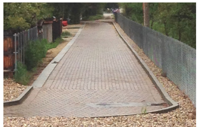
Permeable pavers implemented in an alley retrofit project.
