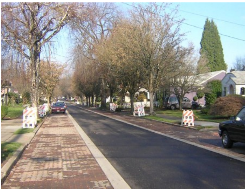
Residential streets can be retrofitted with permeable paving in the parking zone of the street. Source: Nevue Ngan Associates
