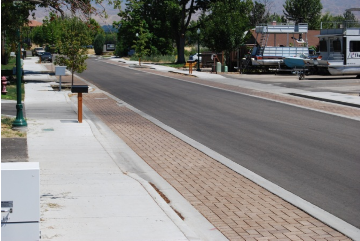
Figure 11. Permeable paver side street parking installed on 36 th Street, Garden City, ID
