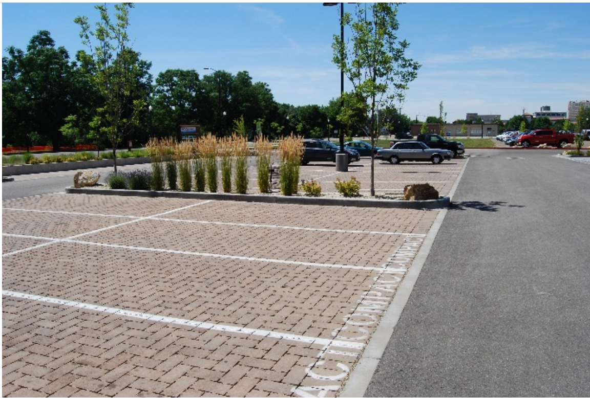
Figure 12. Private interests in Boise have adapted permeable pavement into parking systems
