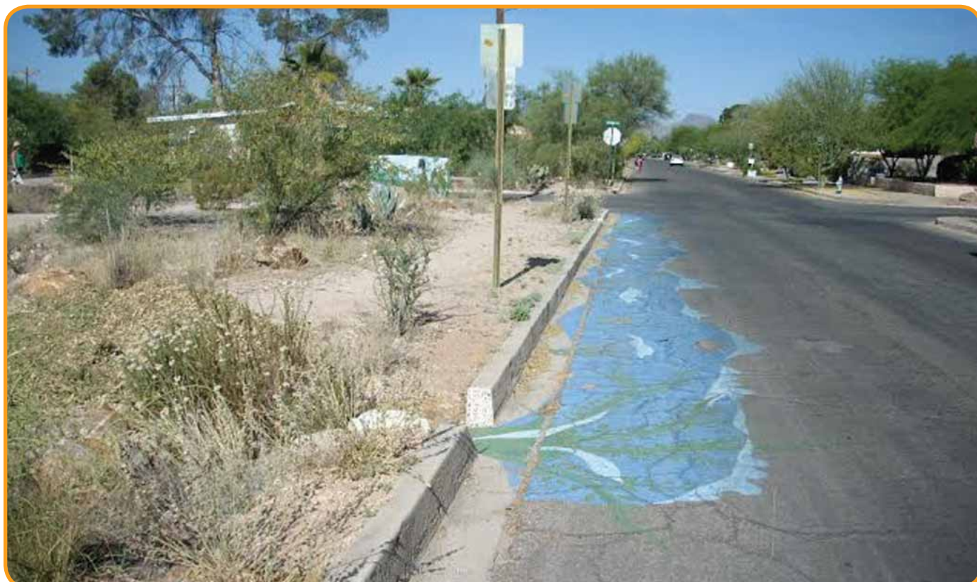
Painted curb cut
