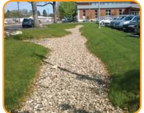
Bioretention Photo by Idaho Rivers United
