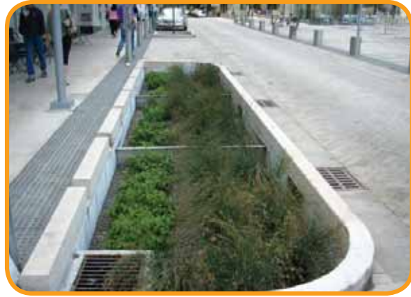
Bioretention Photo by Jeff Adams
