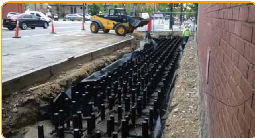
Silva Cell installation
