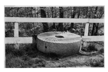
This historic artifact was used to grind grain into flour. There was a waterwheel to power it, that moved a runner stone over a stationary bed stone. Runner stones and bed stones had grooves etched in elaborate patterns, like the bedstone pictured here. The grooves
