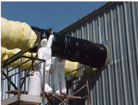
Use Cotton Koozie heat gun to shrink film over insulation.
