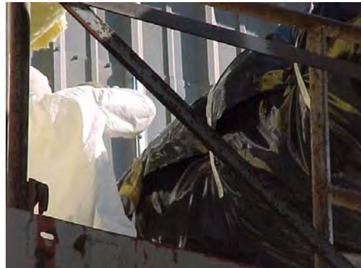
Temporarily secure film with common tape.
