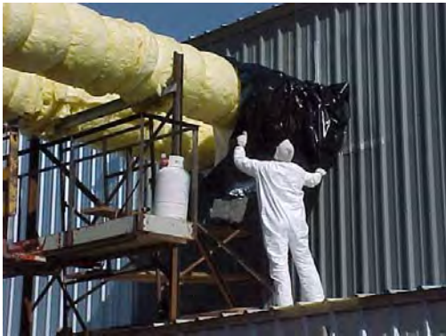
Wrap insulation with film.
