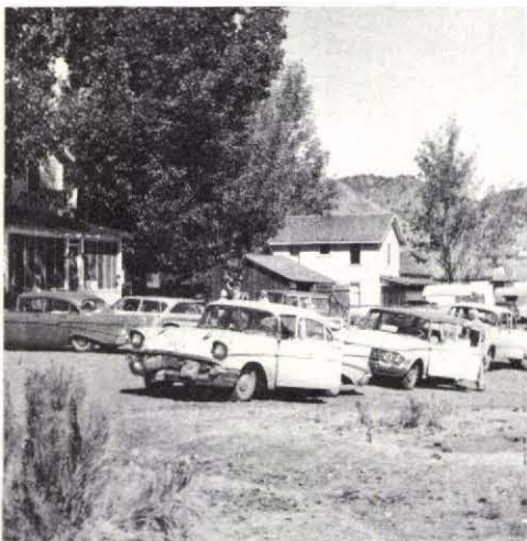
GSOC'er caravan lines up at Frenchglen. (Photo by Delano Photographics.)
