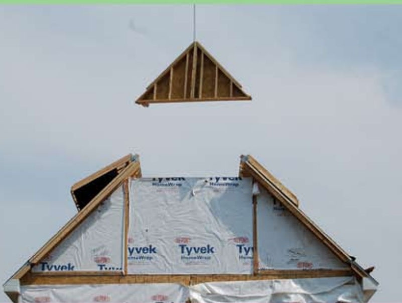
4. The roof sections are set and sealed.
