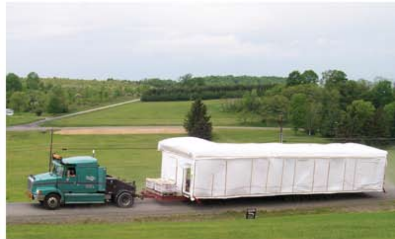
1. Modules are shipped from the factory on super-strength steel carriers.
