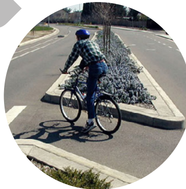
Bicycle refuges in medians provide bicyclists with a much safer option for crossing busy multi lane streets. source: NACTO
