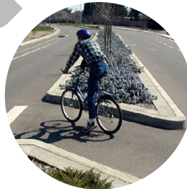
Bicycle refuges in medians provide bicyclists with a much safer option for crossing busy multi lane streets.
