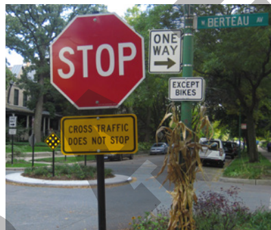
Signage on contraflow lanes should be clearly legible. An "EXCEPT BICYCLES" supplemental plaque should be used in conjunction with all one way signs.
