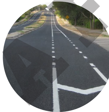
Buffered bike lane in Austin, TX, showing chevron buffer markings and dashed right turn transition source: NACTO
