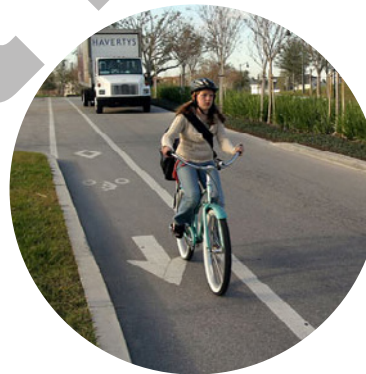
Conventional dedicated bike lane in Baldwin Park, CA, with appropriate roadway markings. source: NACTO
