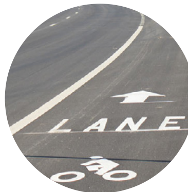
There are numerous options for marking a bike lane, including symbols, words, and directional arrows source: NACTO
