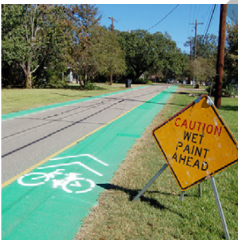
Bike lanes on Capital Heights Ave. were painted to increase visibility and safety.
