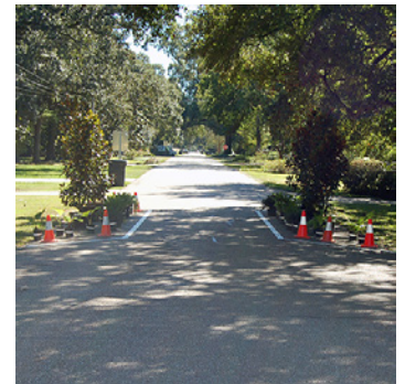
A traffic choker was installed on Richland Ave. to slow down speeding vehicles.
