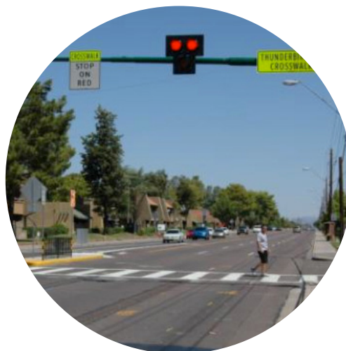
HAWK signal and high visibility crosswalk on a busy street. source: bikepedinfo.org
