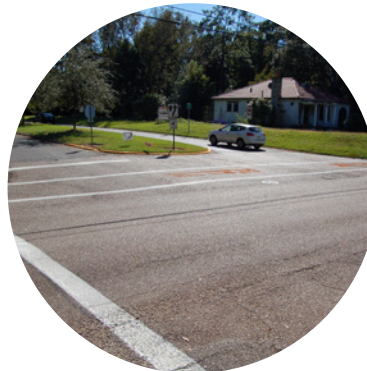
The existing intersection presents a potentially confusing and dangerous crossing for all users. source: CPEX
