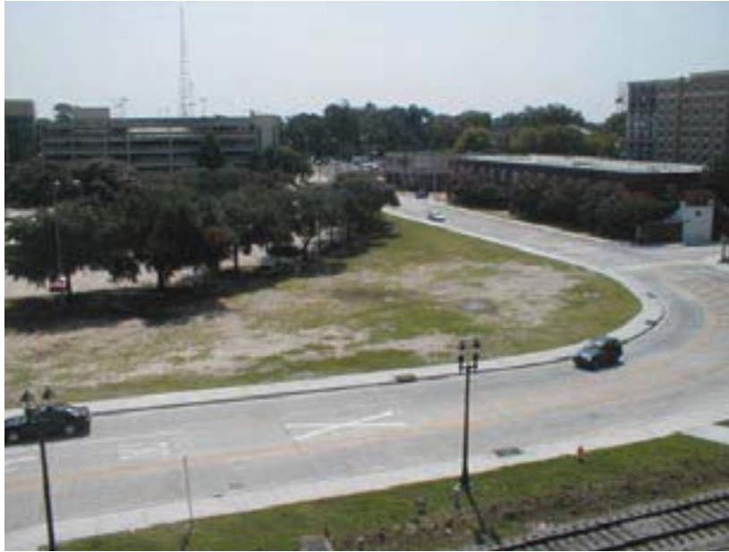
River Road Realignment - Completed May 2002
