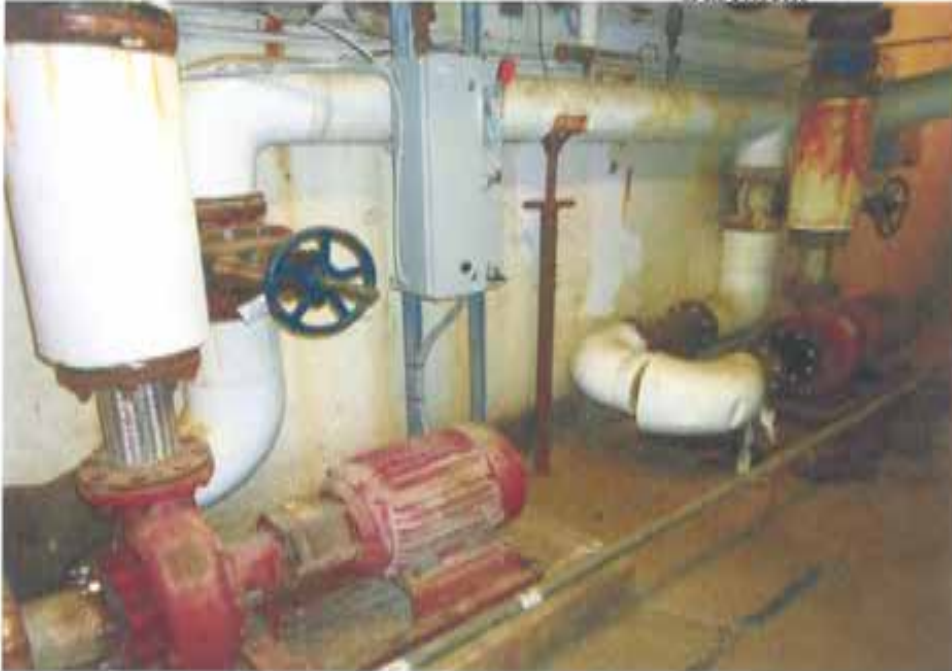
FIGURE M-11: Judson Boiler Room Hot Water Pump (Far left pump has been disconnected) & new condensate pump
