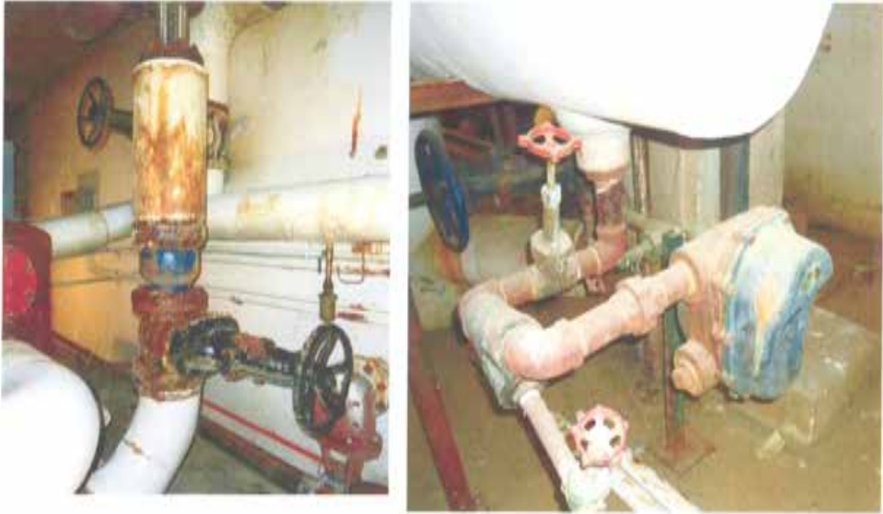
FIGURE M-10: Severely corroded Heating Hot Water & Steam Piping in Judson Tower Basement
