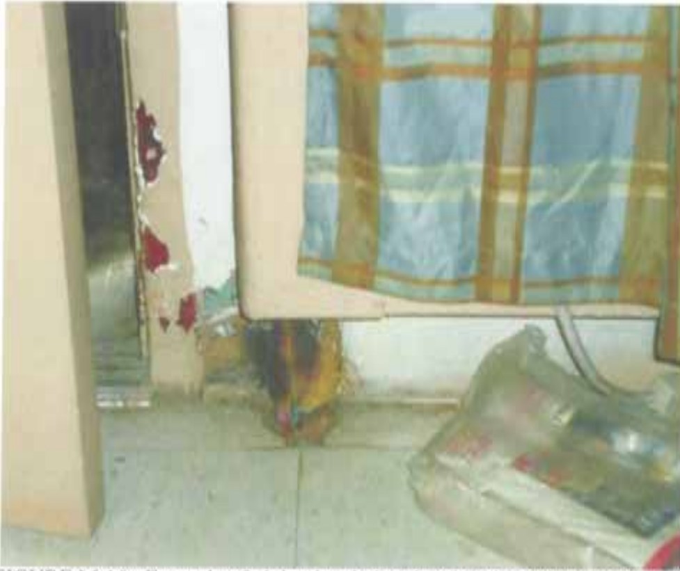
FIGURE M-16: Example of piping insulation deterioration below finned tube radiation convector in high-rise apartment
