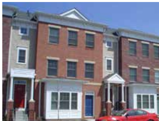
WOODWARD TERRACE, JERSEY CITY, NJ (WRT)
