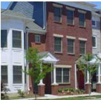
WOODWARD TERRACE, JERSEY CITY, NJ (WRT)
