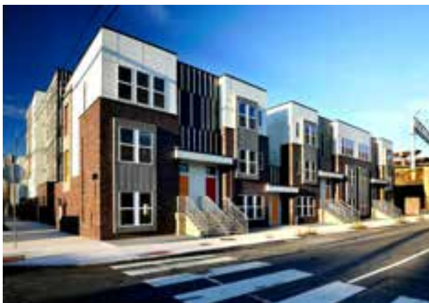
PASEO VERDE (9TH STREET & BERKS STREET) (WRT)
