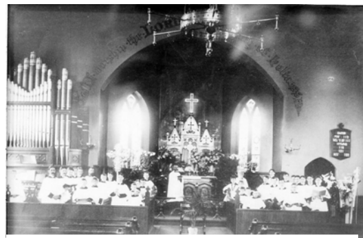
Note gas fixtures.
