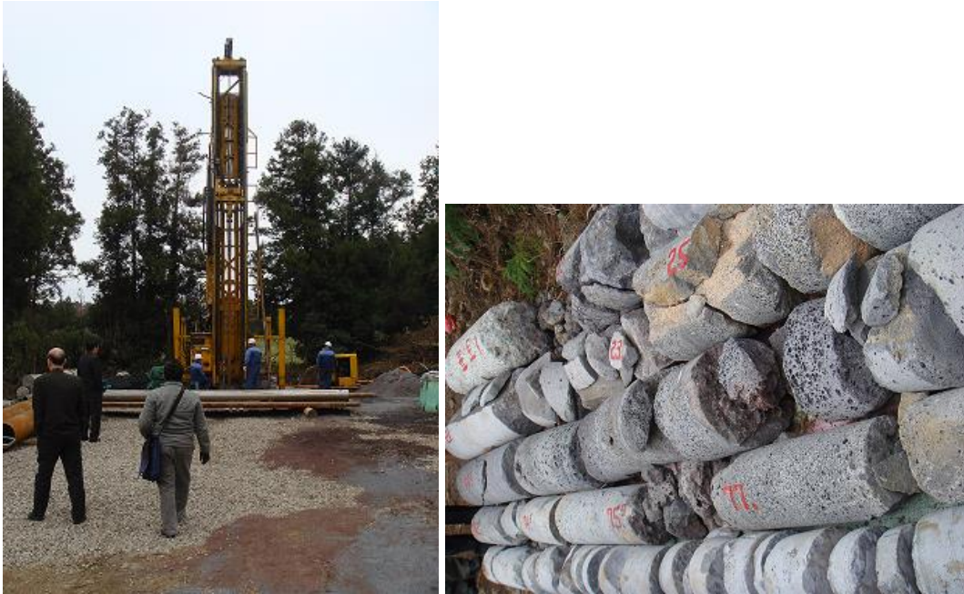
Lateral drilling work (construction process) Ground characterization based on depth
