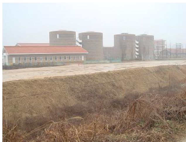
Photo of Daesan Purification Plant
