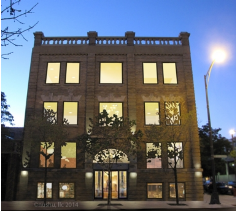
A rendering of a bed and breakfast planned for 1134 W. Washington. Designer: nushu LLC
