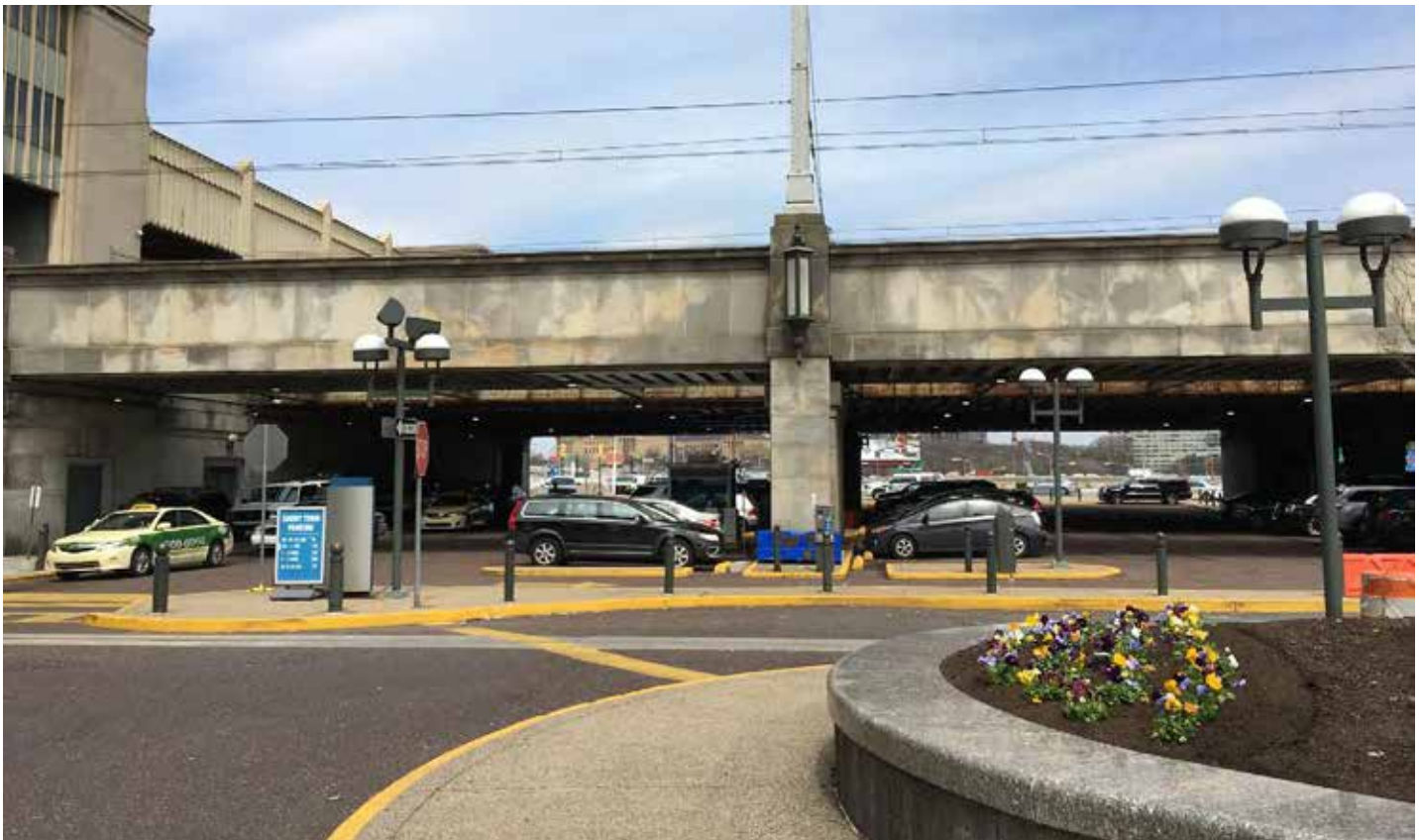
Constrained Parking Under East SEPTA Rail Overpass
