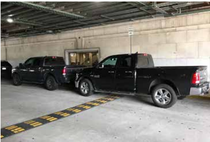
West SEPTA Exit Blocked by Parking
