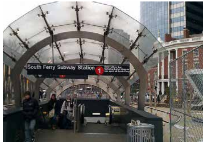
Entry and Exit Point
