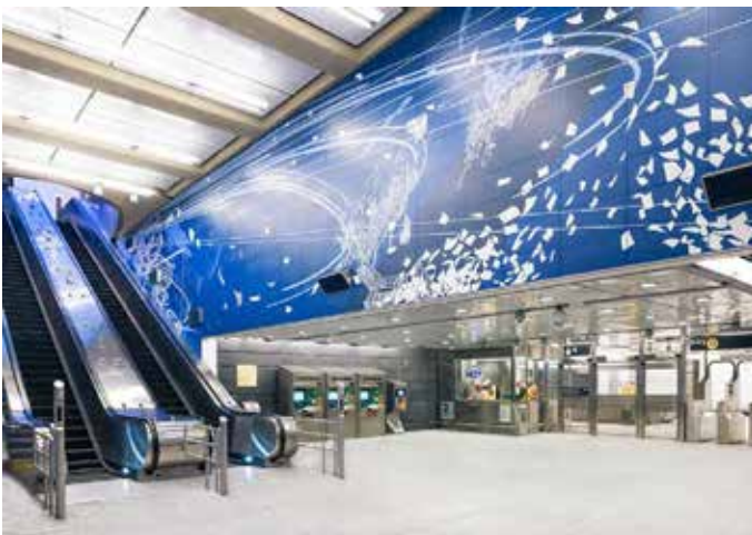
Run Off Space at the End of the Escalator
