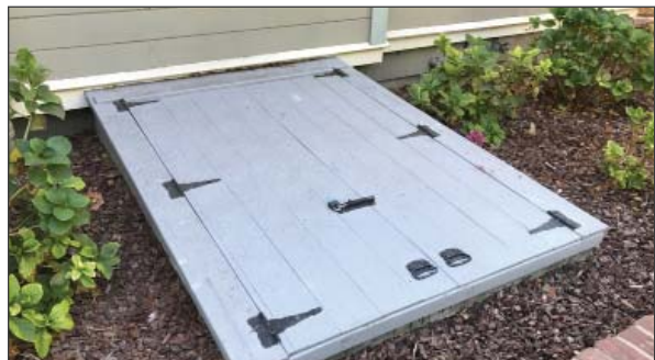
Basement access door. (ARG, 2016)
