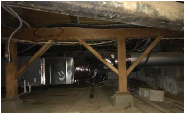
Structural floor framing at crawl space. (ARG, 2016)
