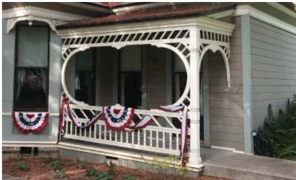
Moon gates and spindle work at northeast porch. (ARG, 2016)
