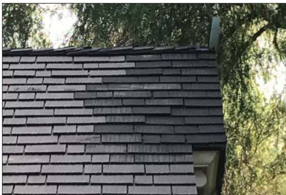
Darker colored tile at east gable end. (ARG, 2016)
