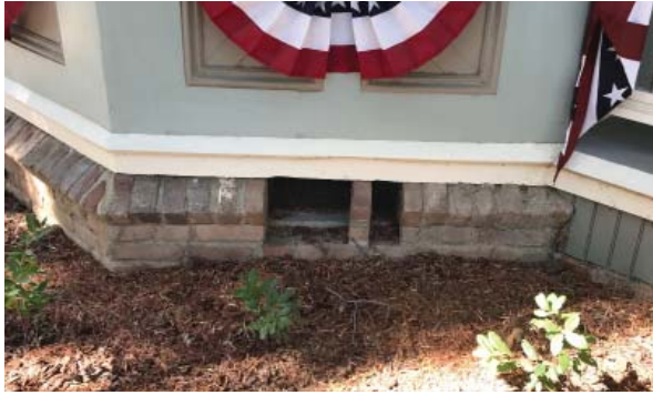
Typical brick foundation and crawl space vents. (ARG, 2016)
