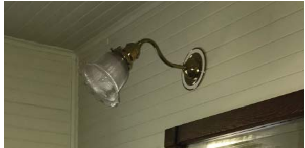
Original wall sconce at master bathroom. (ARG, 2016)
