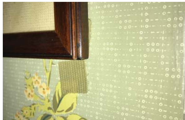
Velcro adhesive at stair hall wallpaper. (ARG, 2016)
