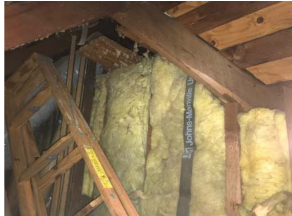
Insulation at attic wall. (ARG, 2016)
