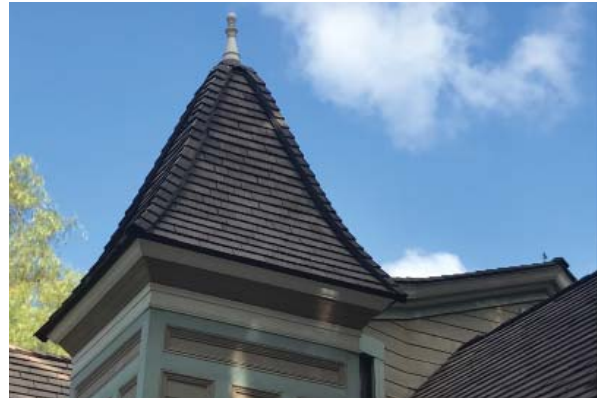
Concrete roof tiles at tower. (ARG, 2016)
