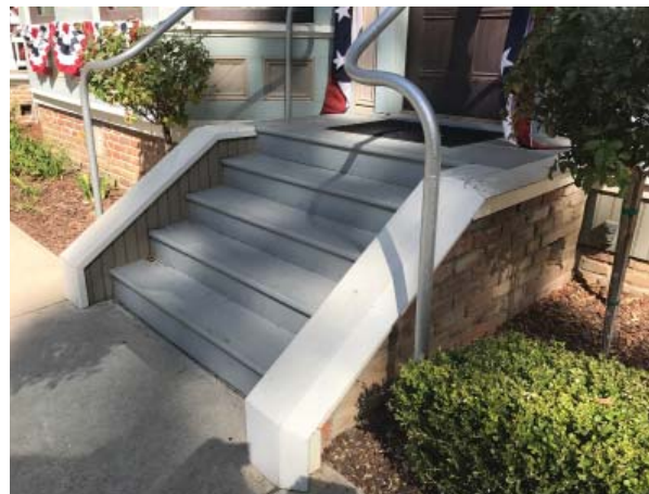
Steps and pipe handrails at main entrance porch. (ARG, 2016)
