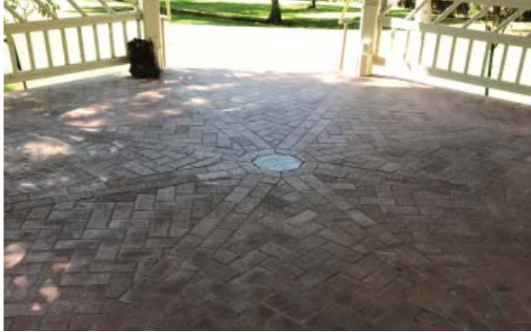
Quarry tile paving and central plaque. (ARG, 2016)
