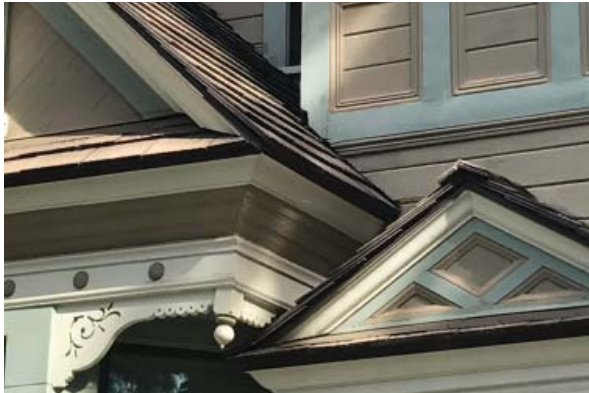
Wood siding and trim details at south elevation. (ARG, 2016)
