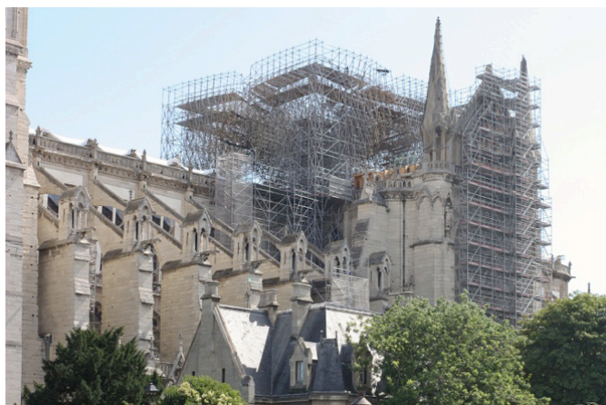
Fig. 5 – Paris, Notre-Dame, restoration scaffolding, July 2019 (photo: Lindsay Cook).
