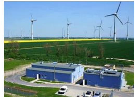
P2G project in Grapzow, Germany
