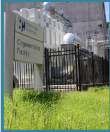
FuelCell Energy power plant at Hartford Hospital
