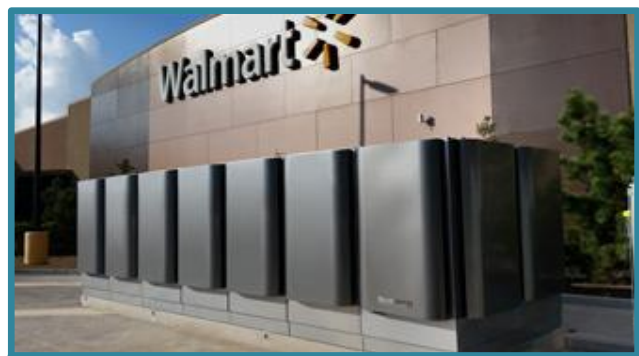
Bloom Energy fuel cell server at a Walmart retail site
