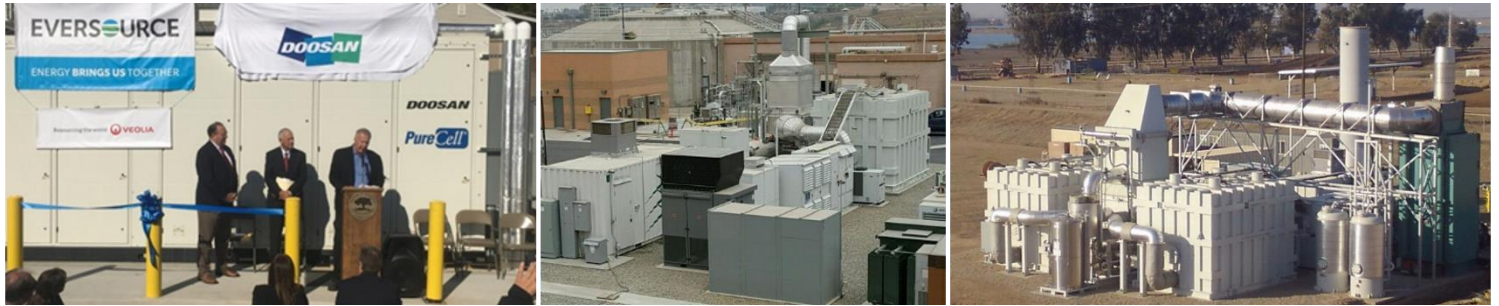
Figure 2. Doosan Fuel Cell America fuel cell at Naugatuck WWTP in Connecticut (L). FuelCell Energy fuel cell at Riverside WWTP in California (C). FuelCell Energy fuel cell at Tulare WWTP in California (R)
