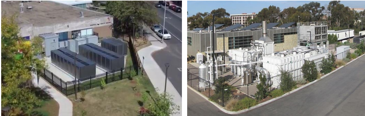
Figure 1. Bloom Energy fuel cell microgrid in Hartford, Connecticut (L). Microgrid with FuelCell Energy fuel cell at UCSD (R)
