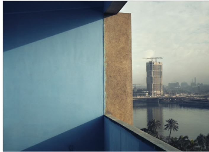
Adam Bartos, Cairo, Egypt (Ramses Hilton under construction) , 1980, pigment print, 31½" x 41½". Gitterman.
