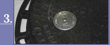
Place badge in flat area of cover, taking care to ensure it is positioned properly before pressing down to bond mastic to cover. Open cover and push bolt through hole in badge, mastic pad and hole in cover.
