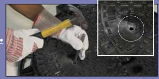
With cover closed, punch through hole in center of flat area
