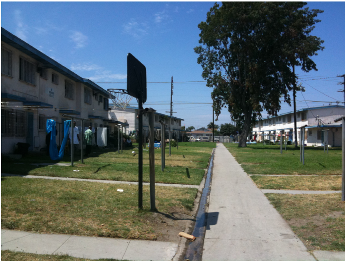
Jordan Downs Housing Project, Watts, CA
