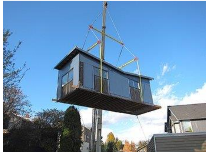
ADU lowered into a backyard.
