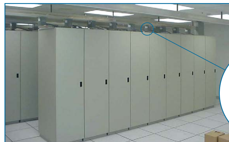
STARLINE puts a full access track busway overhead for a clean appearance, dramatically improved accessibility, and much less risk of human error during changeover or addition.
