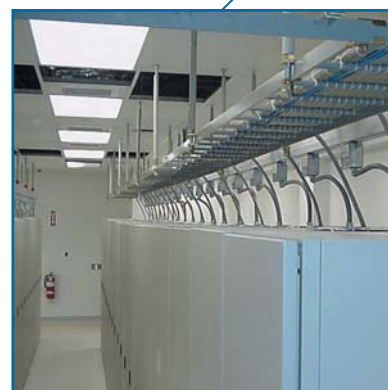
Circuit protected power modules can be supplied with multiple NEMA outlet devices, drop cords or hard wired to each cabinet as needed.
