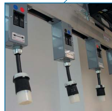
Each power module is circuit protected with fuses or circuit breakers right at point-of-use.
