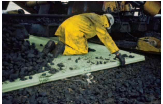
Fig. 9: Laying of Styrodur C into the track bed.
