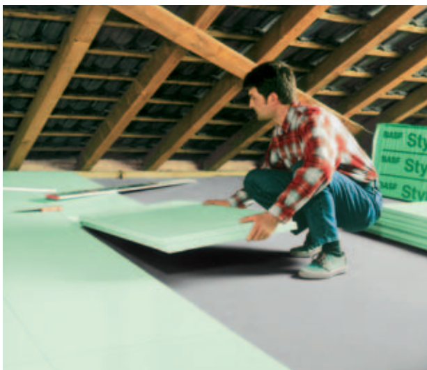
Fig. 10: Insulation of an attic with Styrodur® C.
