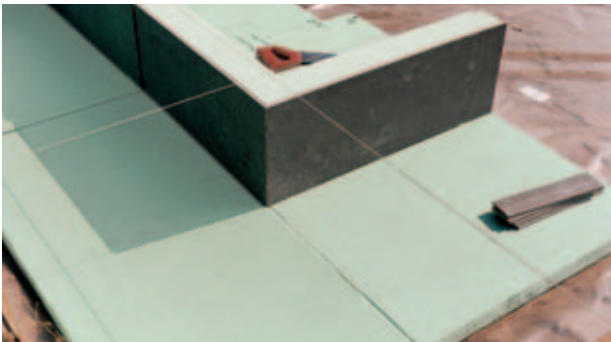
Fig. 3: Insulation of a foundation slab with Styrodur® C.
