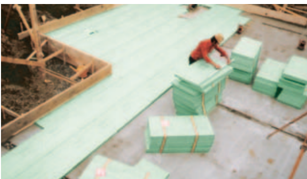
Fig. 4: Laying of Styrodur C boards.
