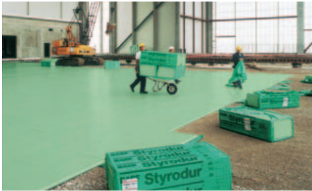
Fig. 23: Insulation of industrial floor with Styrodur® C.
