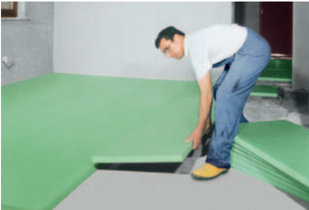
Fig. 19: Insulation of basement floor.
