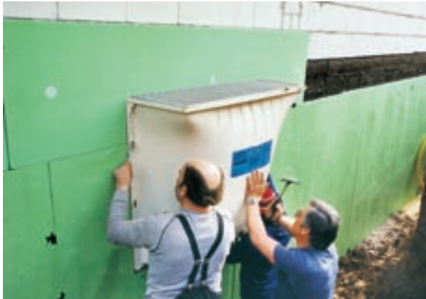
Fig. 3: Perimeter insulation with Styrodur® C.
