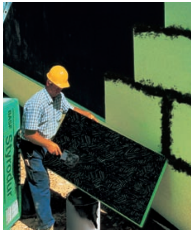
Fig. 25: Adhesion of Styrodur® C boards (full surface & edges) and plastering of the grooves for boards installed in groundwater.
