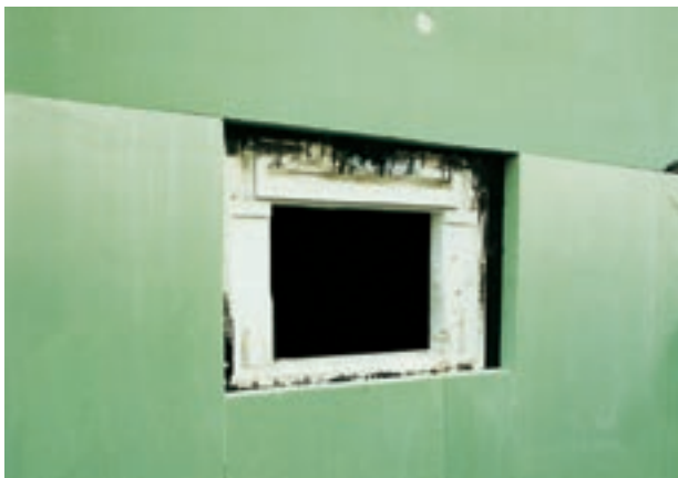
Fig. 4: Insulation measures with Styrodur® C.
