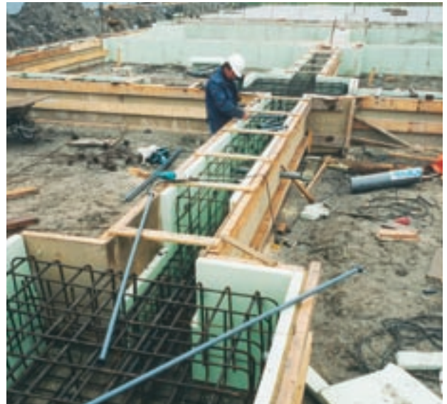
Fig. 15: Formwork with Styrodur® C.
