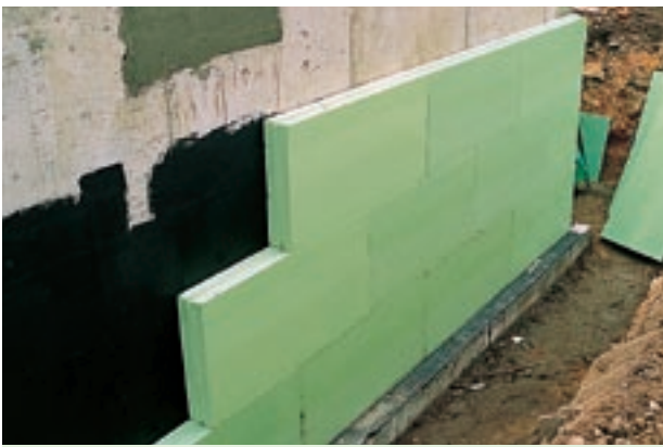
Fig. 5: Conjoined installation of Styrodur® C boards.
