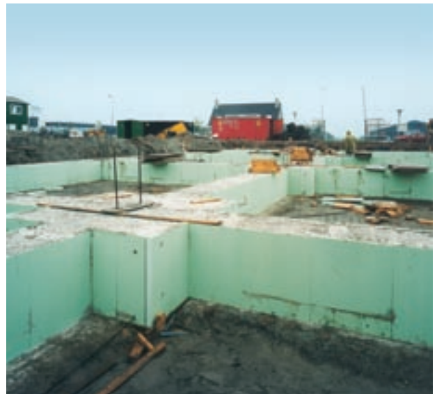
Fig. 16: Styrodur® C boards installed into formwork.
