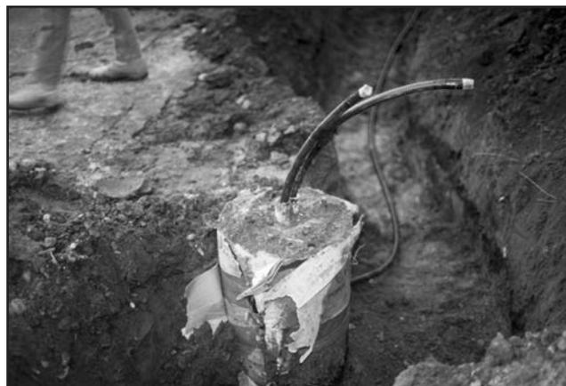
Figure 5.3.2—PVC Jacketed Cable (courtesy AFC Cable Systems)
