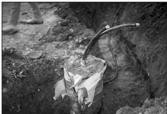
Figure 5.3.2—PVC Jacketed Cable (courtesy AFC Cable Systems)
