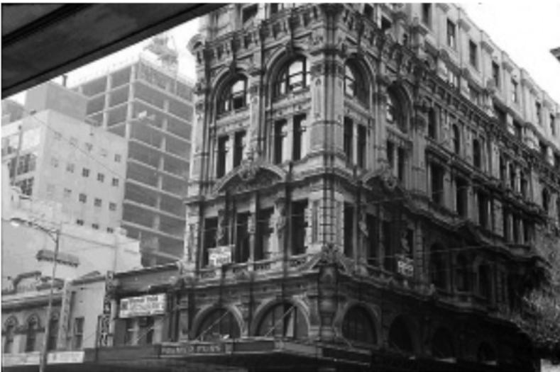
Melbourne Town Hall Chambers, cnr Swanston and Little Collins Streets, demolished 1968. Photo: K.J. Halla, SLV.
