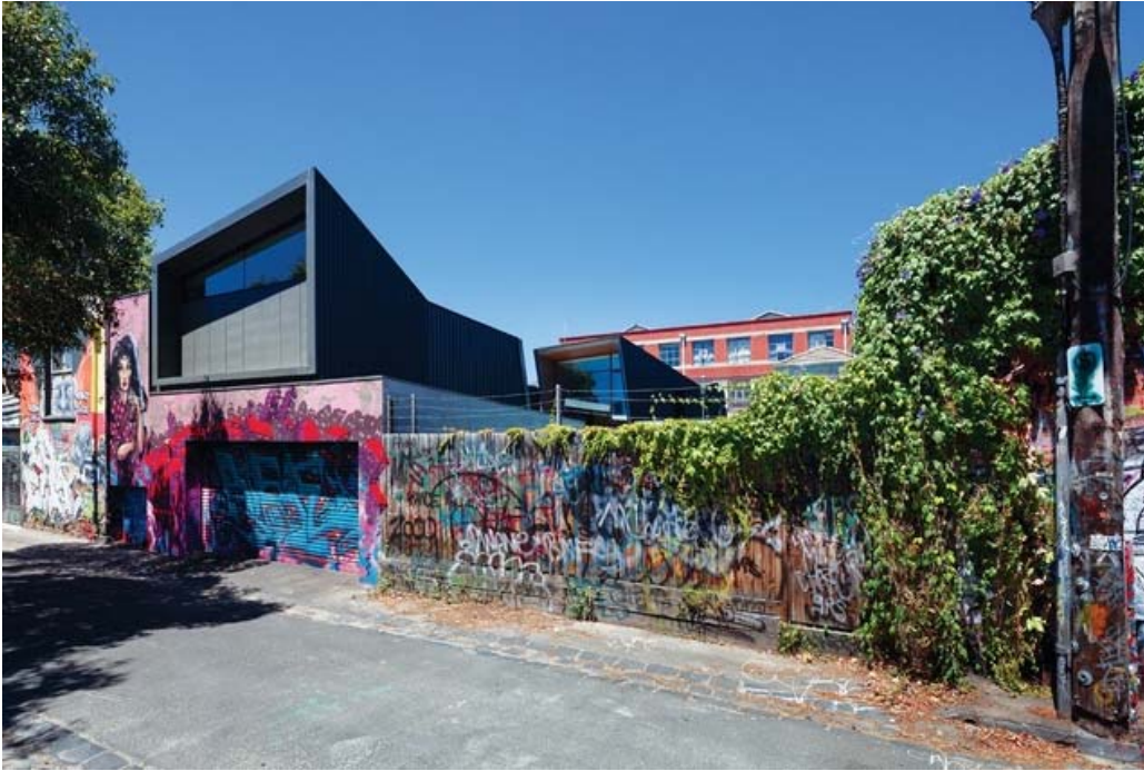
The two pavilions “find their alignment” in a view to a gum tree. Image: Trevor Mein
