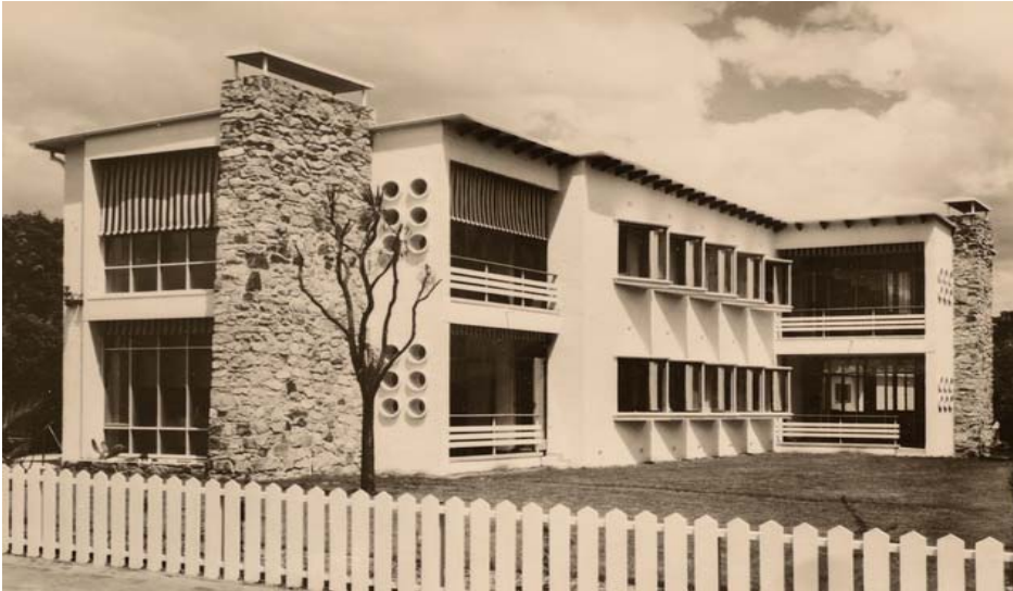
Romberg and Shaw, Glenunga Flats Armadale, 1940.
