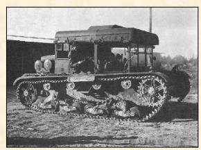
C7P tractors were used for towing 220mm wz.32 Skoda heavy mortars, and also acted as recovery vehicles for light tank companies. The C7P was also used by some engineer units.
