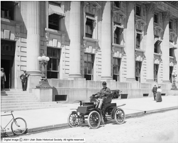
Post Office and Courthouse Building* 1908
